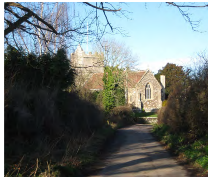
fig. B. The church seen from where Church Lane meets the village edge.
