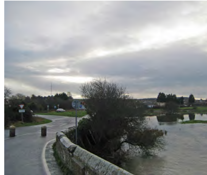
1. View south towards Wool from the original historic bridge over the River Frome.
