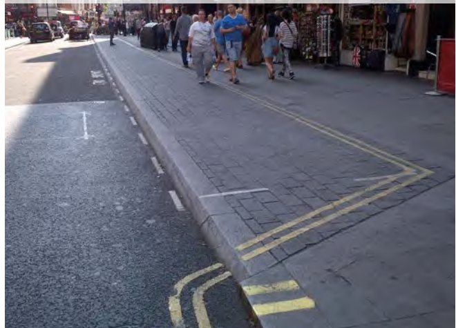
Figure 7.11: Inset loading bay ensures that carriageway remains 'narrow' to reinforce low speeds and provides space for pedestrians.
