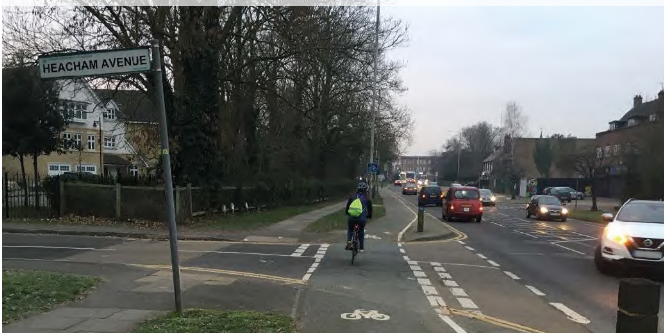
Figure 10.16: Partial set back, marked priority crossing, Hillingdon
