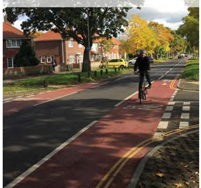
Figure 6.21: Centre line removal, Norwich
