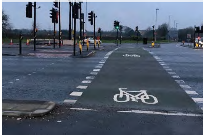
Figure 10.9: Single-stage straight-over cycle crossing next to multi-stage staggered pedestrian crossing, South Gloucestershire
