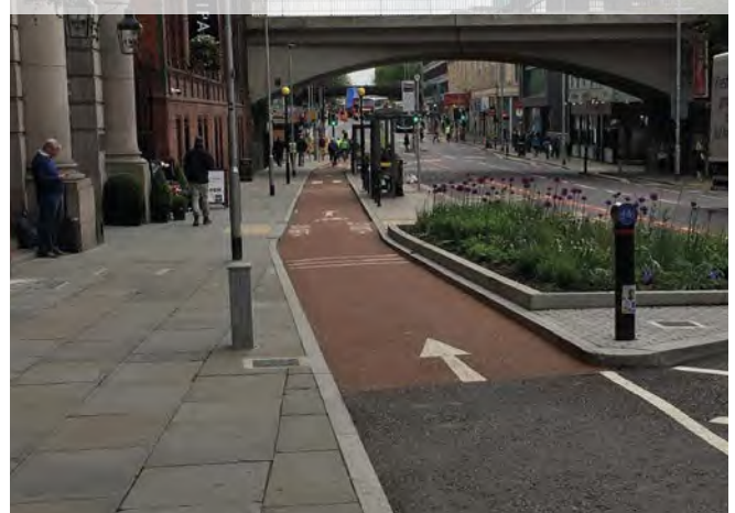
Figure 9.4: Cycle lane to cycle track transition
