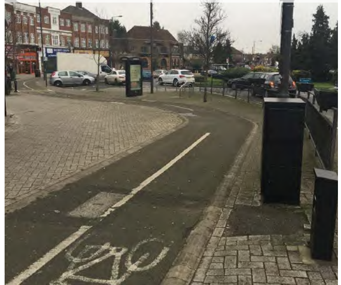
Figure 10.36: Footway-level cycle track around large roundabout, Harrow
