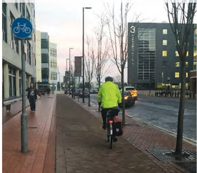
Figure 6.14: Cycle track with sign to TSRGD diagram 955
