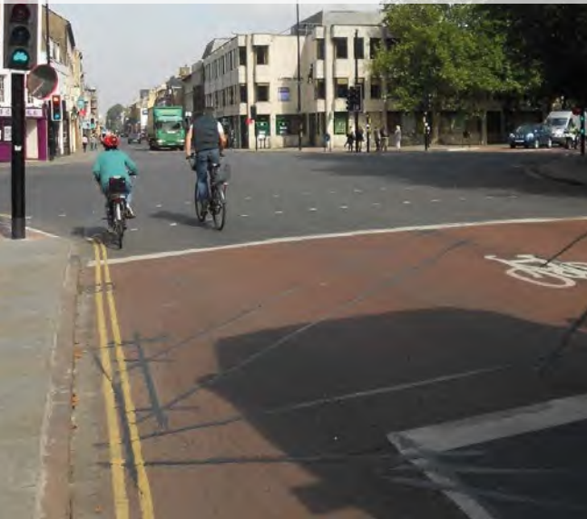
Figure 10.23 'Cycle Filter' signal used for an early release, Cambridge
