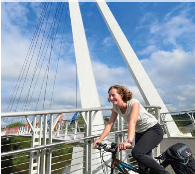
Figure 10.49: Diglis Bridge, Worcester
