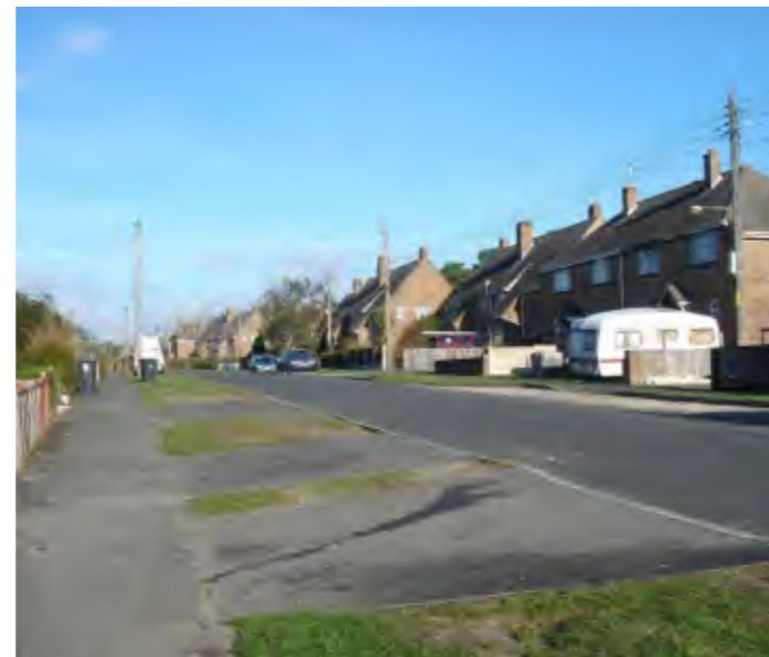
2. The various residential estates generally have standard estate roads as here at Cologne Road.
