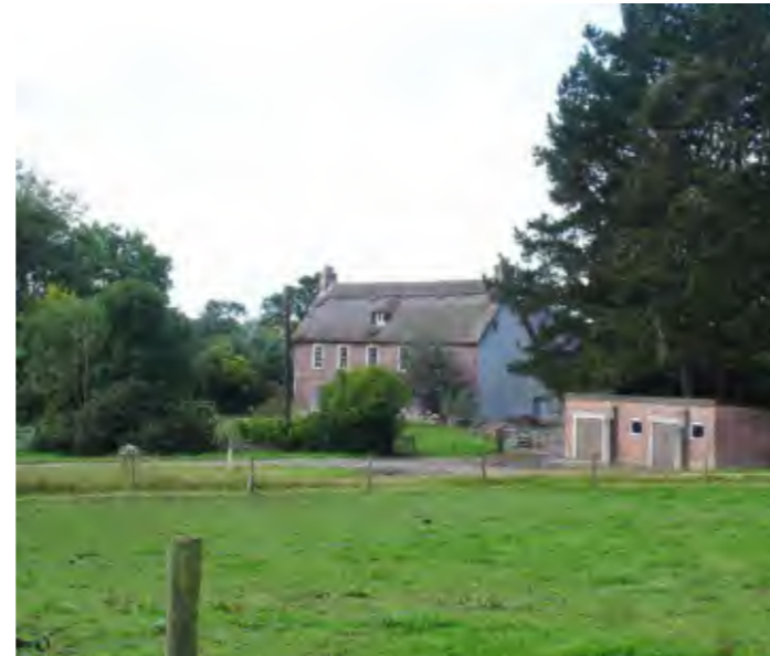
1. Bovington Farm predates the military camp and was part of a complex of farm buildings that has since been demolished.
