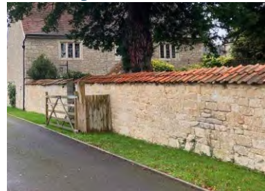
(2) red barrel tile-capped stone, of a rough course
