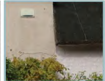
Light coloured render including thin render over a stone wall.
