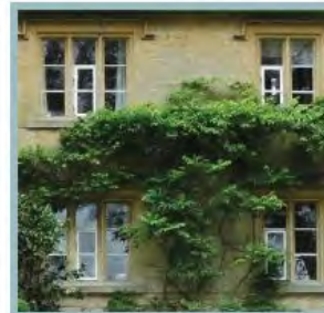
Casement window with chamfered stone mullions.
