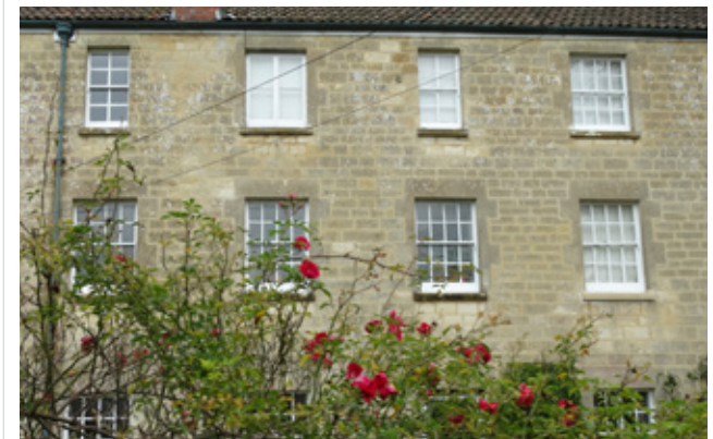
Figure 30: Well-proportioned and placed sash windows that are slightly setback into the facade and feature glazing bars.
