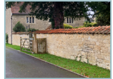
Red barrel tile capped stone wall that is of a rough course
