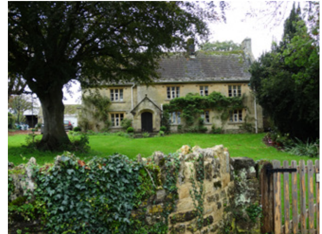
Figure 06: Example of a coursed square rubble facade.
