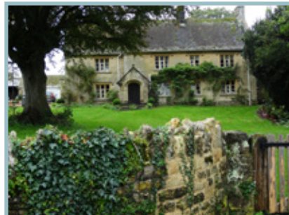
Stone wall with lime mortar topped with larger 'cock and hen' cap stones
