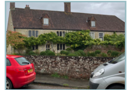
Mid-rise brick wall capped with a thin, flat mortar
