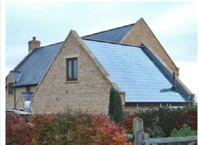
Figure 46: Solar panels should be integrated into the design of buildings from the outset. This example of a new home in a Conservation Area shows how the panels can mimic the appearance of traditional slate roofs.
