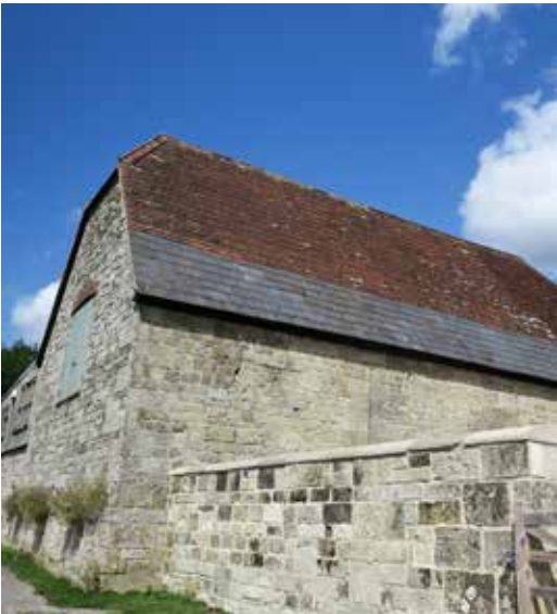
Manor Farmhouse barn: half hip roof with clay plaintile and slate cladding.
