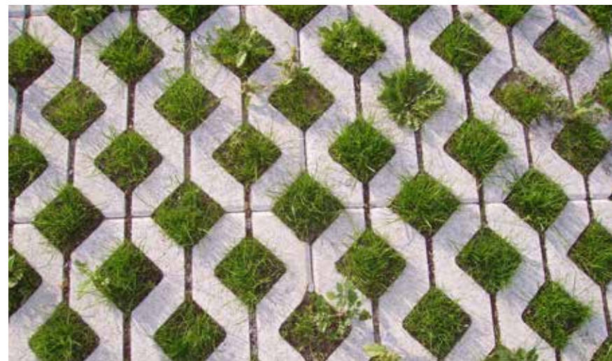
Figure 51: Examples of permeable paving (© Wikimedia Commons).
