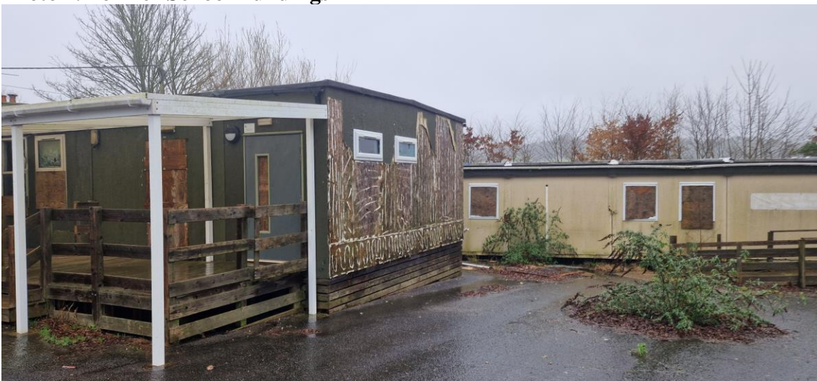
Photo 1. Former School Buildings
