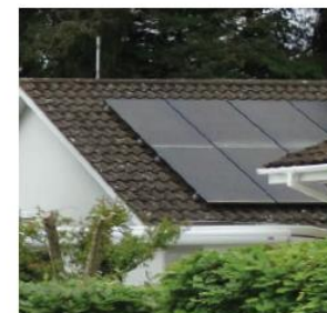
Roof solar panelling.
