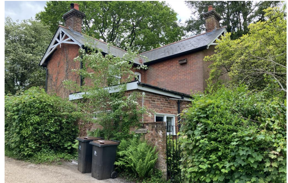
Figure 13. Decorative gable end, ridge tiles and chimneys
