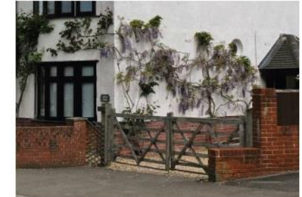
Low brick wall with timber entrance gate.
