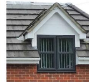
Gable dormer with painted timber casement window.
