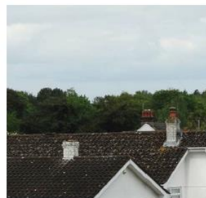
White painted chimneys placed closer to the street scene.
