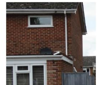
Satellite dish pushed back from the street scene.
