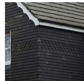
Continuous pattern in weatherboards and decorative fascias.
