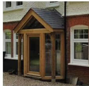
Gable portico with timber frame and glazing.
