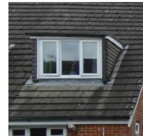
Flat roof dormer with casement windows.
