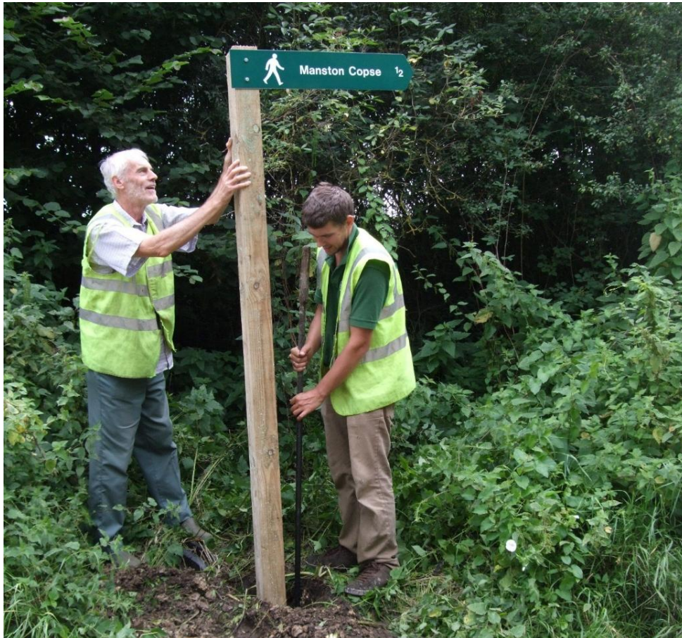
Figure 8: Staff member and a volunteer installing a 'priority sign' in north Dorset.
