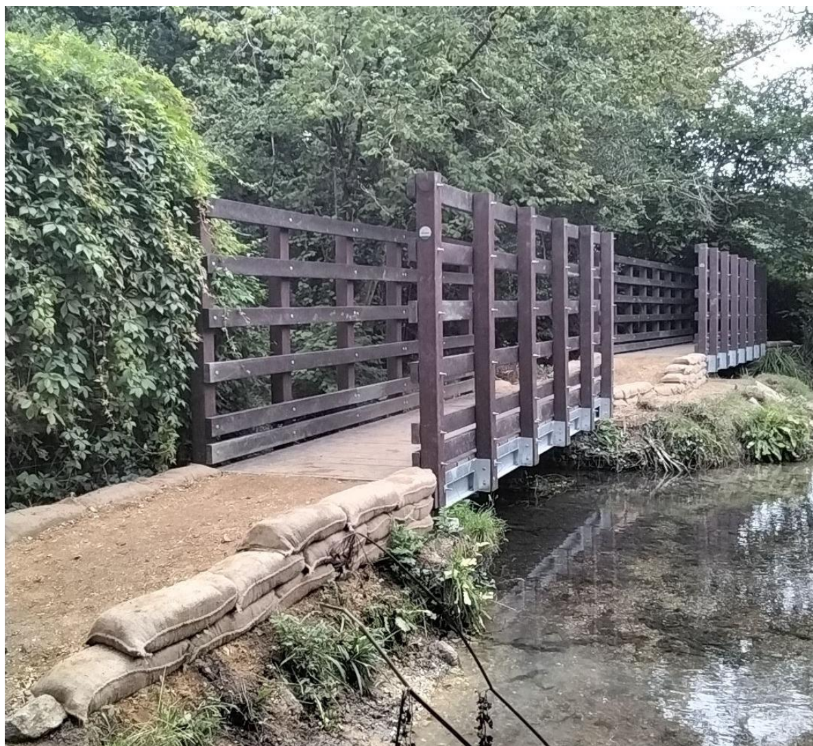
Figure 5: Two recycled plastic bridleway bridges installed near Broadmayne, with sandbag headwalls forming a gentle, step-free ramp to improve accessibility for all users.
