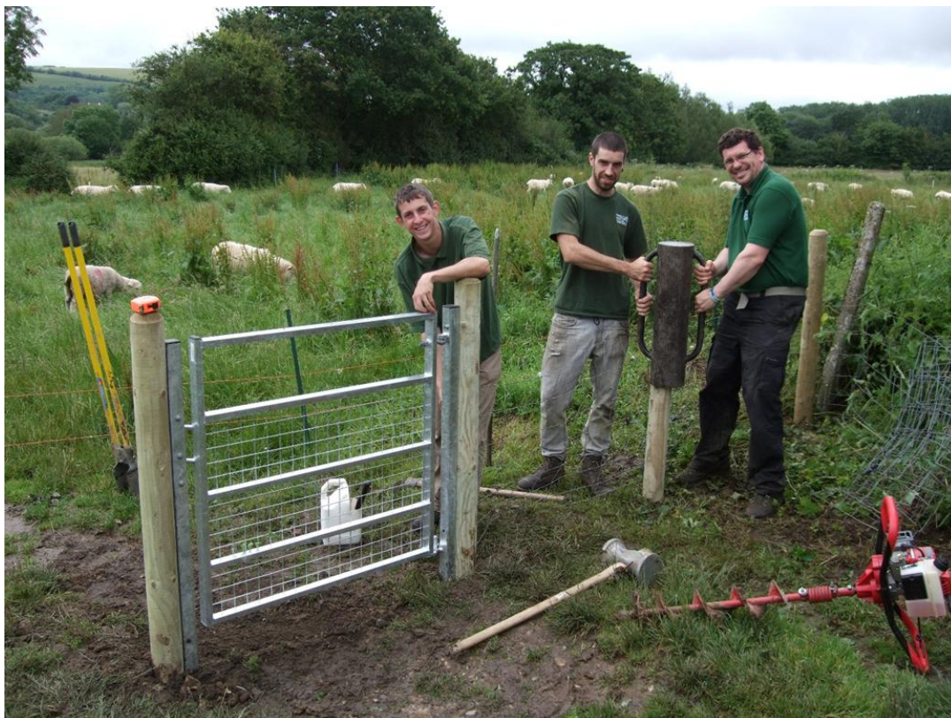
Figure 4: Staff and volunteers installing a new, accessible, self-closing gate.
